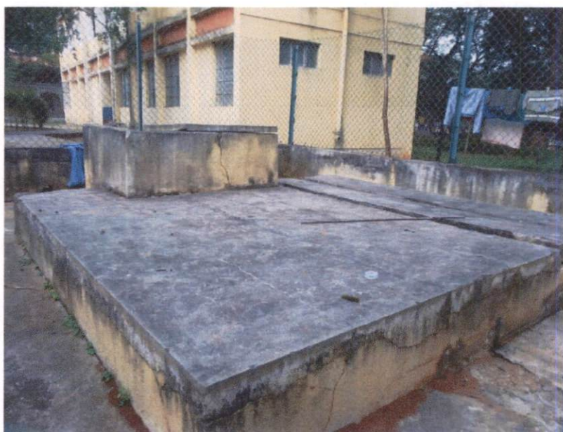
Water storage Sump behind Block-III boys hostel
