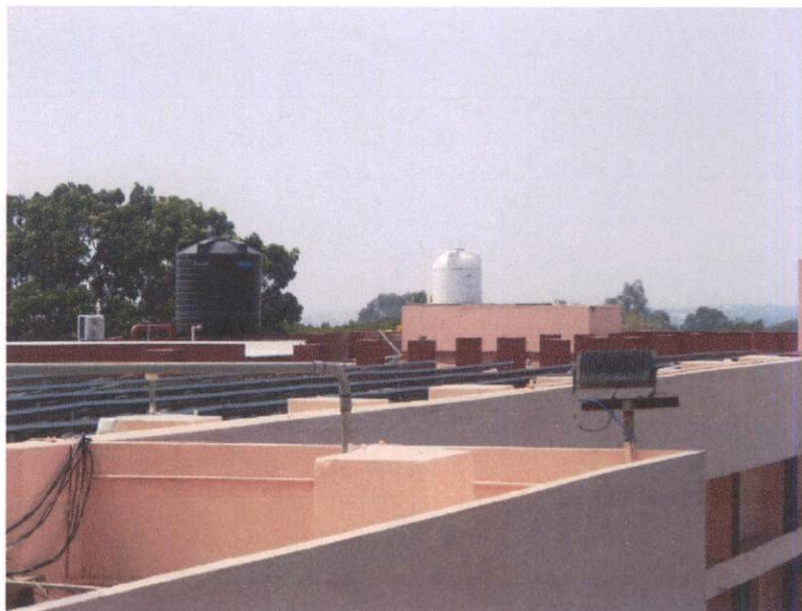
Overhead water storage tank (Admin Block)
