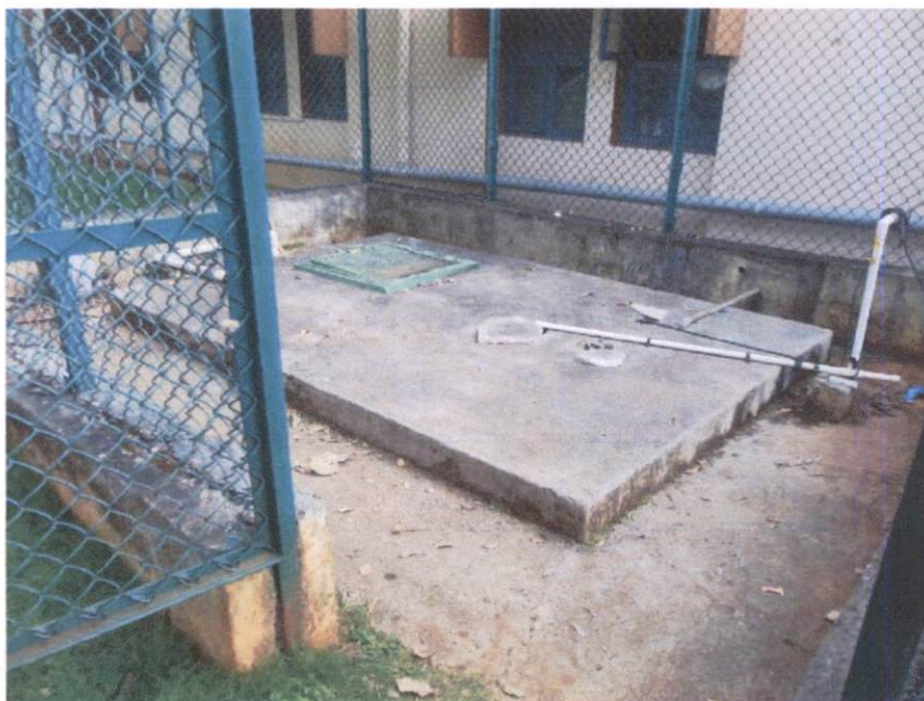
Overhead water storage tank located at boys hostel (block III)
