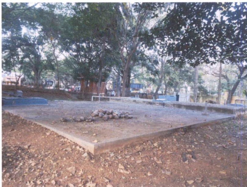
Overhead water storage tank (Gym)
