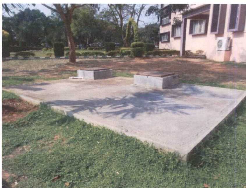
Underground Sump CMS Backside
